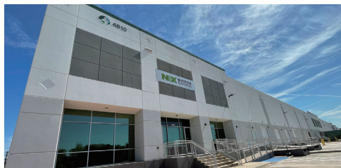
New warehouse in San Antonio, Texas
